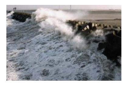
Figure 1.1: Wave run-up and overtopping at Zeebrugge breakwater during (mild) storm conditions (from OPTICREST project, awww.rug.ac.be/opticrest).
