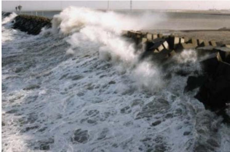
*Figure 1.1: Wave run-up and overtopping at Zeebrugge breakwater during (mild) storm conditions (from OPTICREST project, [www.rug.ac.be/opticrest](http://www.rug.ac.be/opticrest)).*
